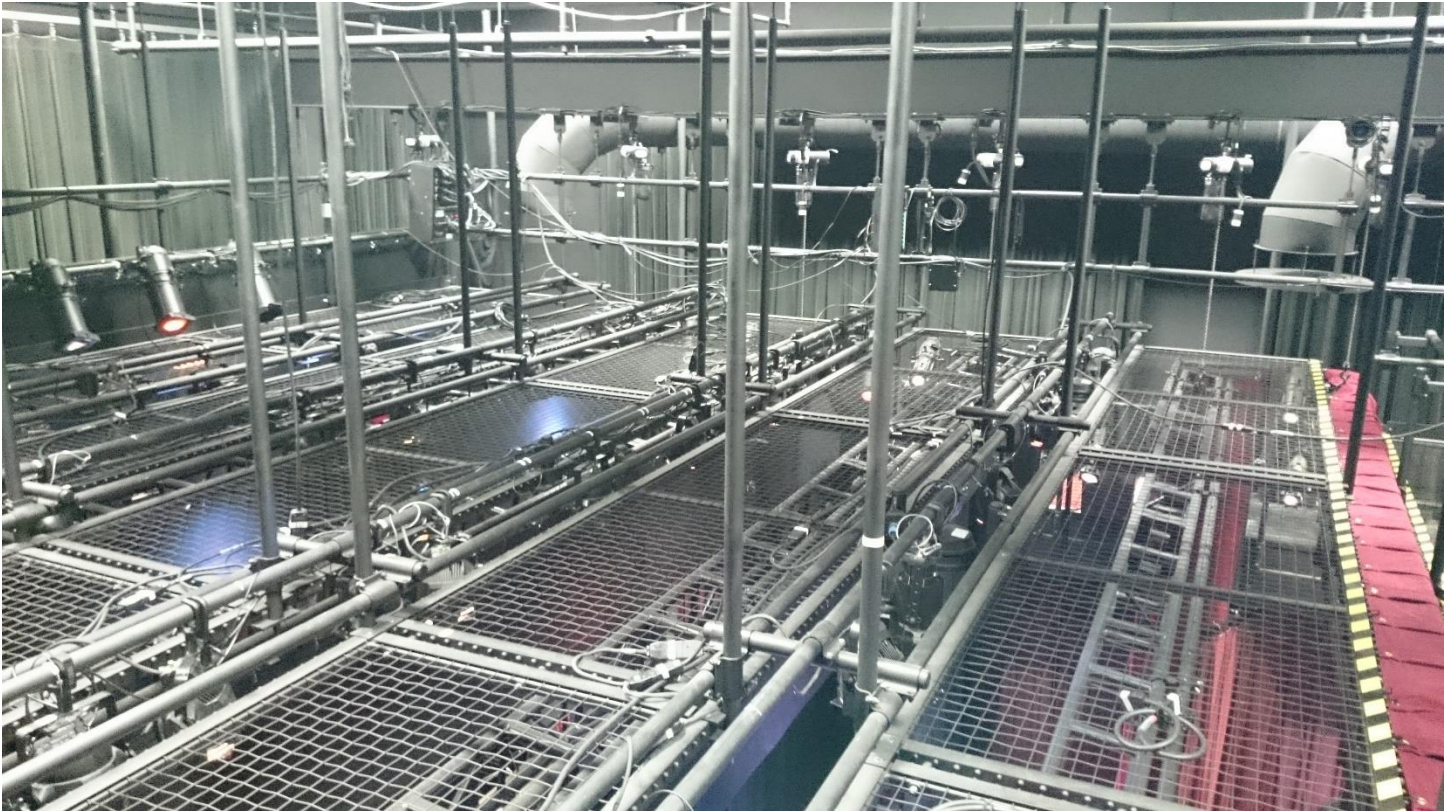
Lighting grid over stage.
