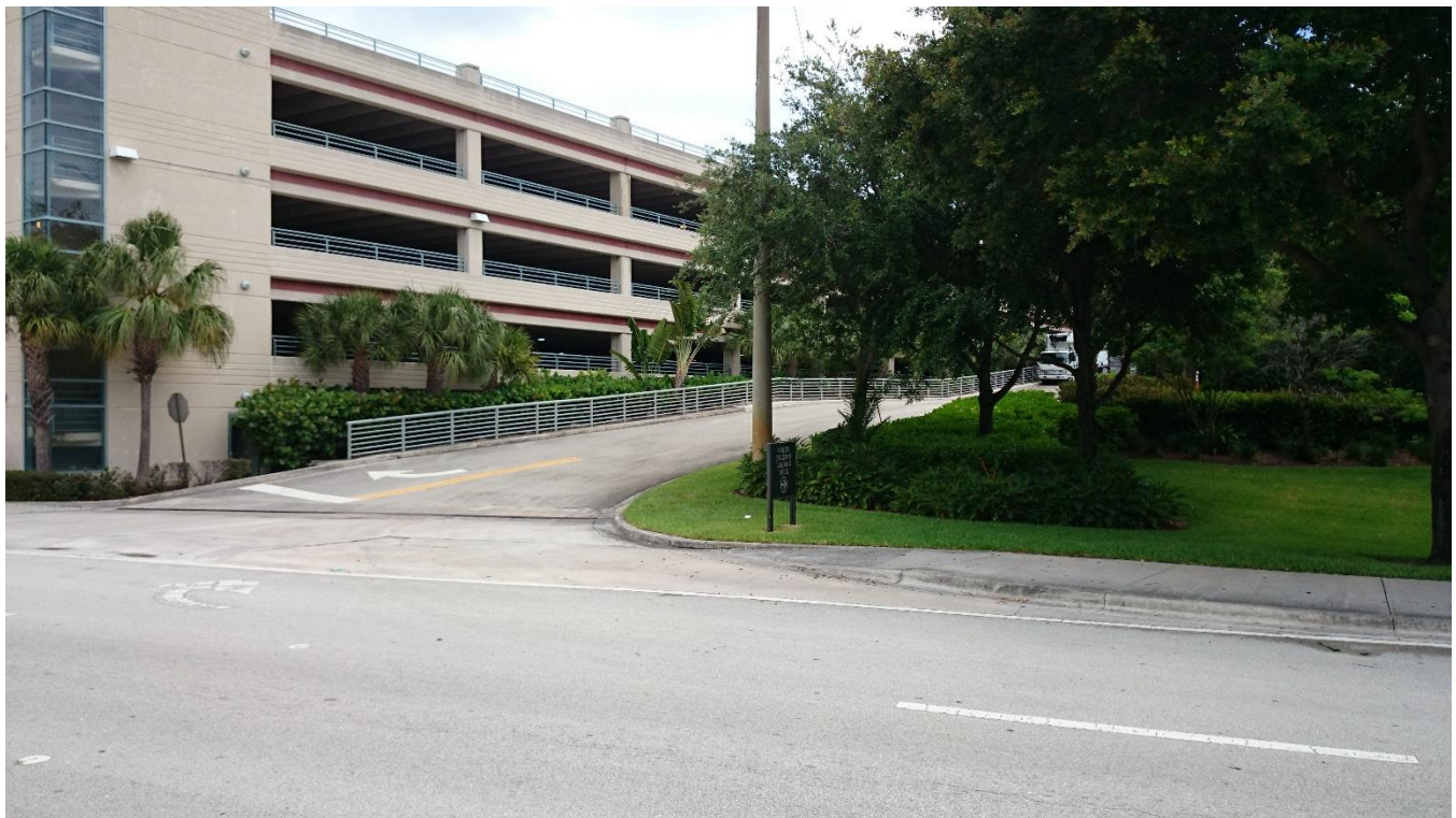
View of truck ramp to Cohen loading dock. Turn BEFORE the parking garage.
