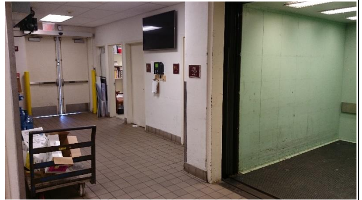
Corridor from loading dock to elevator.
