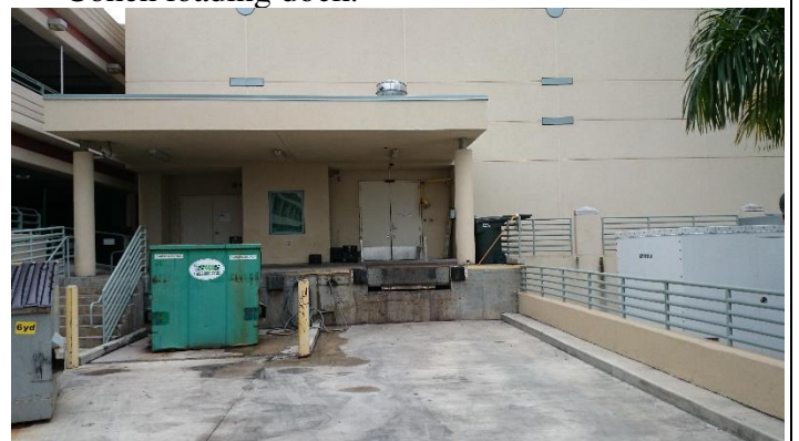
Cohen loading dock.
