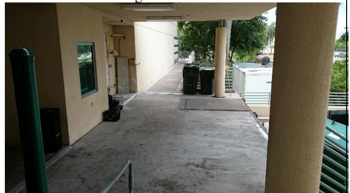
Cohen loading dock.
